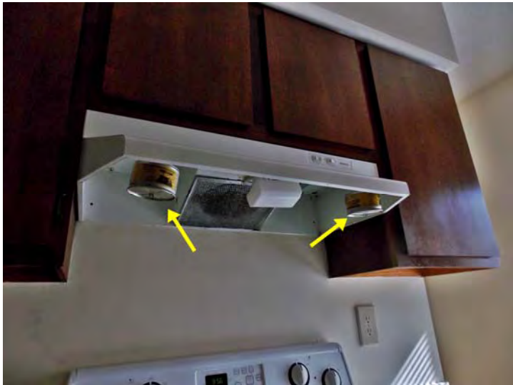
Portable fire extinguishers are included in each rangehood.
