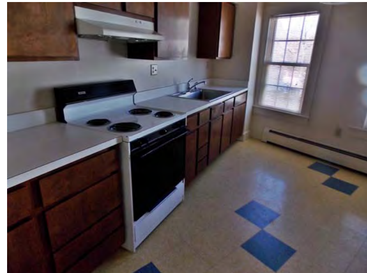
Kitchens include plywood cabinets, laminated particleboard countertops, electric ranges, and VCT flooring.
