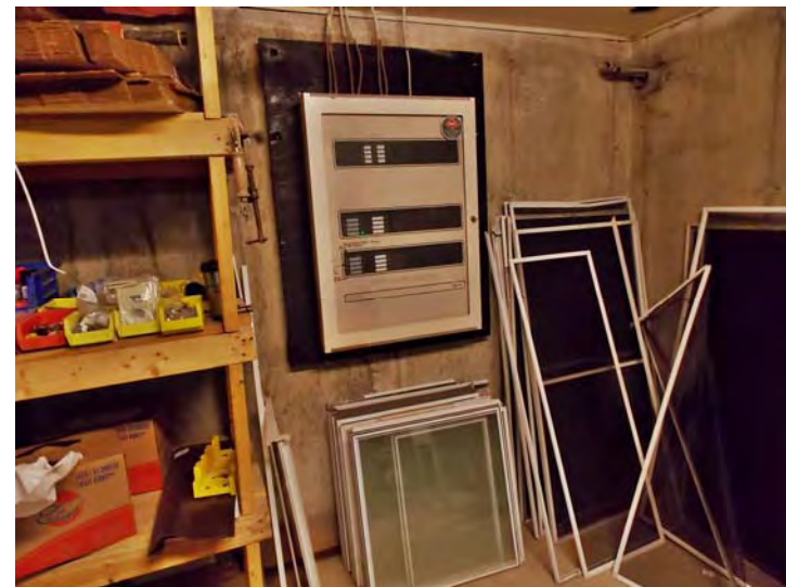
This is the central fire alarm control panel (FACP).
