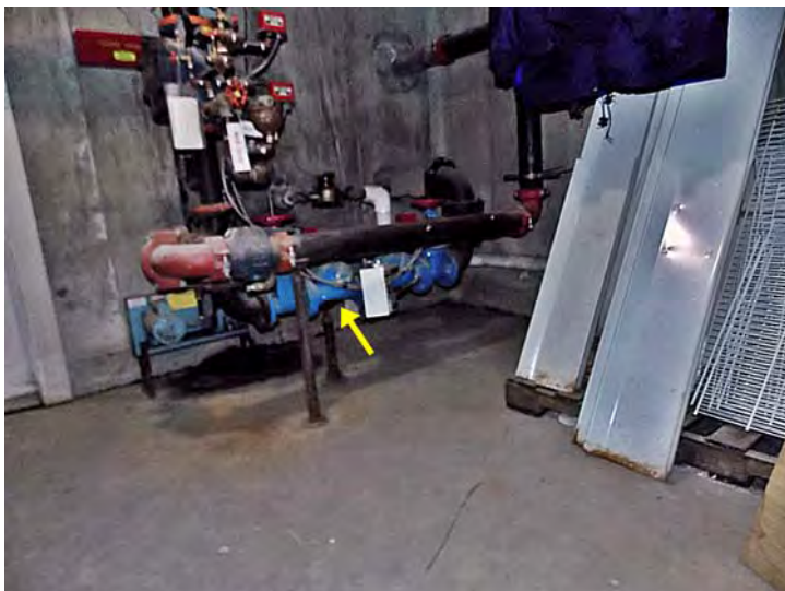
The fire sprinkler connection (serving the Office building) includes a backflow preventer (blue).
