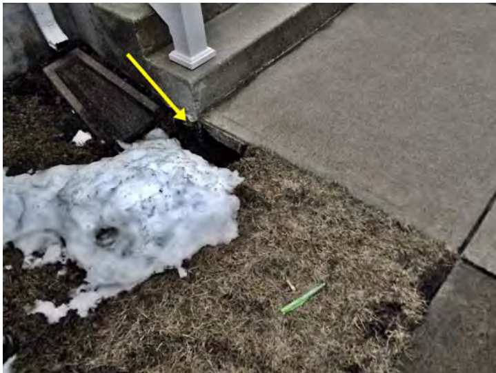
Localized erosion near a building entrance.
