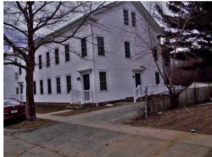
The residential buildings are similar in design and configuration; each has a pitched roof, vinyl siding, single-glazed windows and most have six-panel doors.
