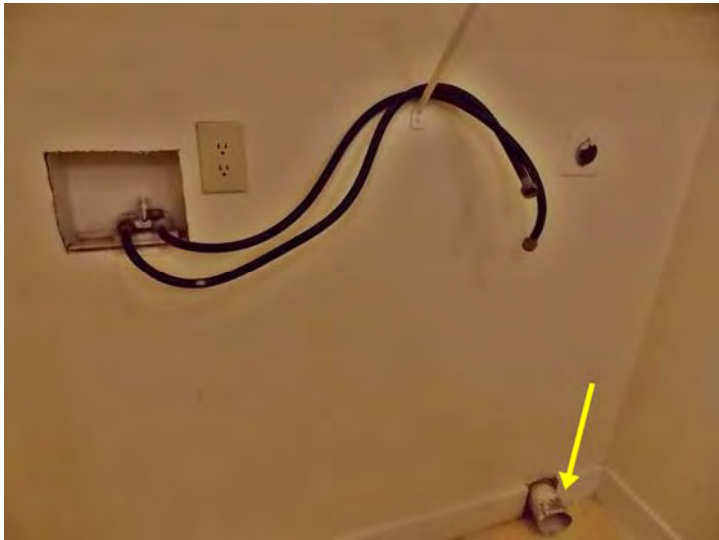
One of the washer/dryer hookups within an apartment. The dryer vent is on the lower right (arrow).
